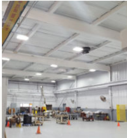
Central Maintenance Shop AFTER
